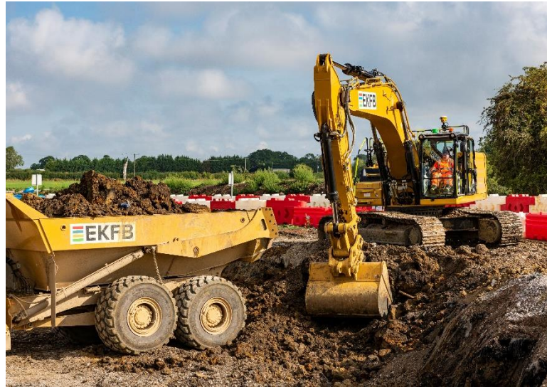
Continuation of Earthworks
